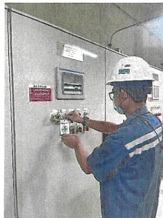
Local Operator "Off" lube oil system function และ "Off" Fuel gas comp.21
